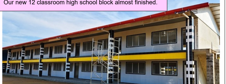
Our new 12 classroom high school block almost finished.
