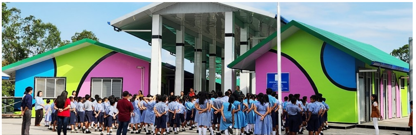
Lining up to start a new school week in our fabulous renovated primary school. What an incredible blessing.
