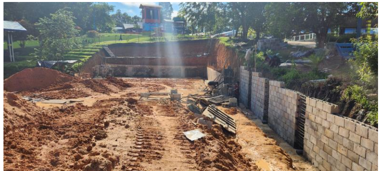
Levelling the area and building retaining walls for the new 6 class room primary (elementary) school building.
